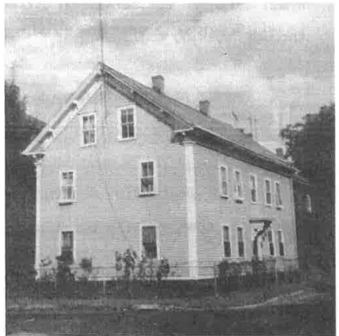
Worker's house - 26 Lafayette Street
