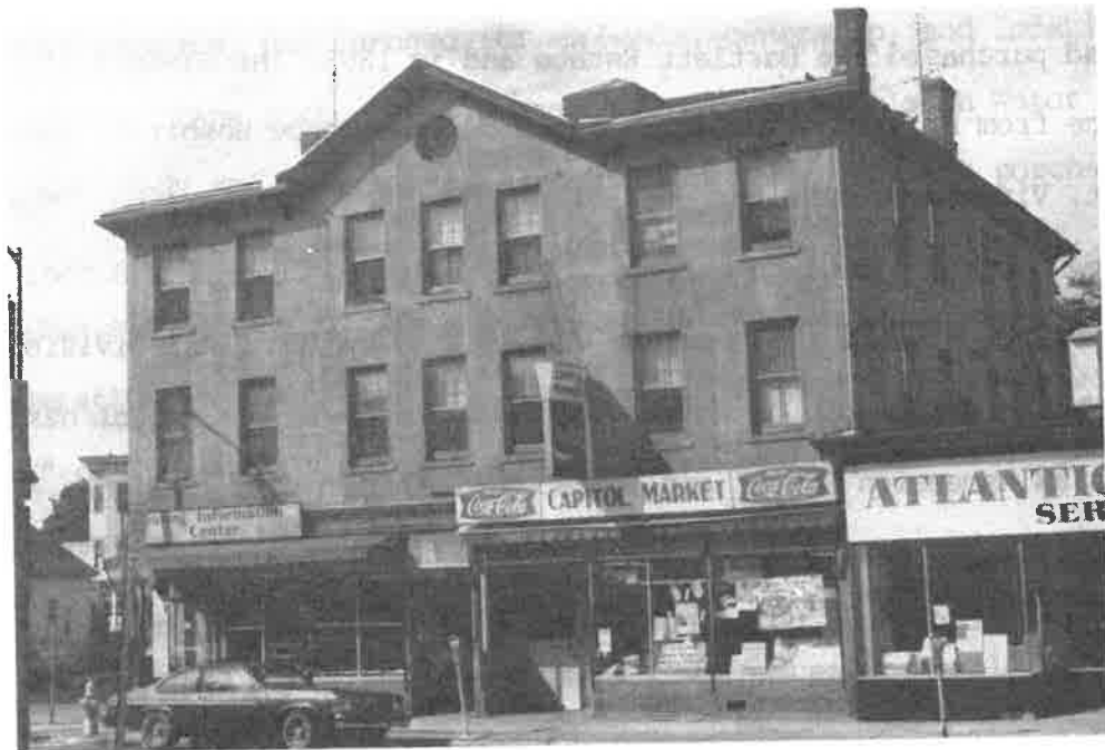
Comstock Building - 118-122 Millbury Street
