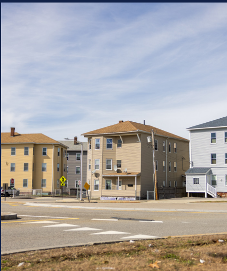
Mill Brook Conduit, a tunnel for water installed in 2007, runs beneath this rotary on Olde Millbury St.
