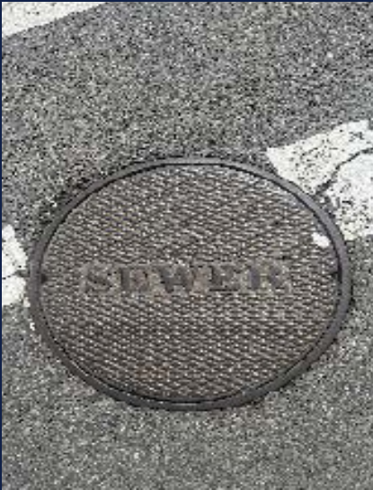
Maintenance hole on Harding St. leading to Worcester's combined sewer system
